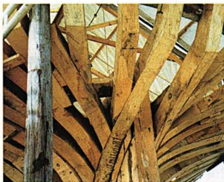
The stern being rebuilt in new timber.
