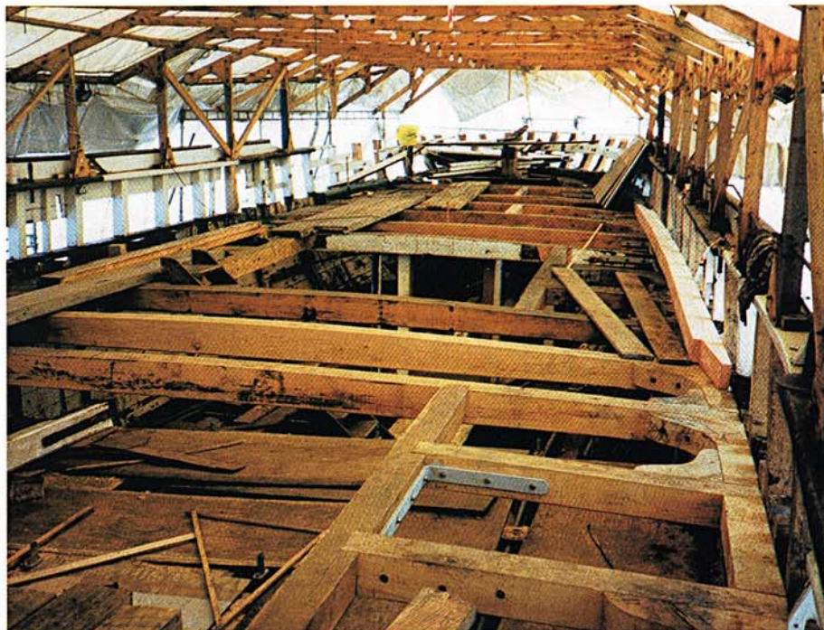
The newly-fitted beams that were to support the deck timbers.
